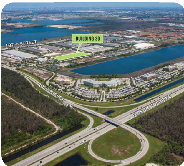
Building 30 (rendering, right) is Flagler Station's newest industrial development.
